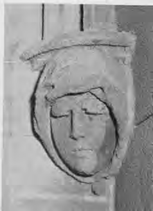
Corbels at South Side Entrance Exterior stone weather-beaten
