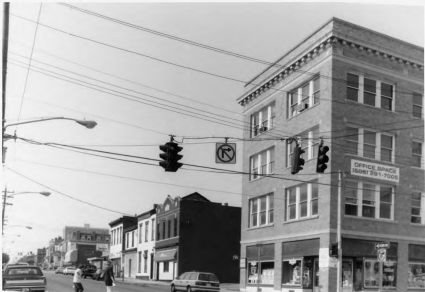
Covington Downtown Commercial Historic District (expansion) Kenton Co. 124 1
