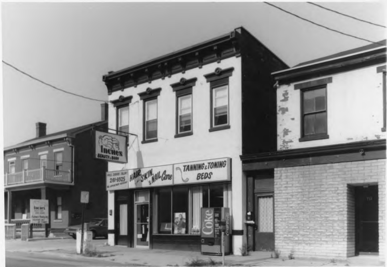
Covington Downtown Commercial Historic District (expansion) - 2014
