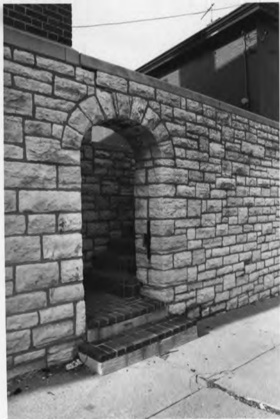
detail at rear of St. John's; Lewisburg Hist. Dist.; Kenton Co., KY
