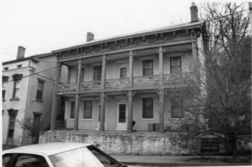
901 Western Avenue; Lewisburg Hist. District; Kenton County, KY
