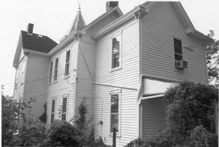
Metcalfe-Stephens House Kenton Co., Ky photo 4
