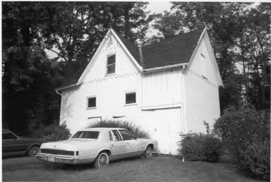
Metcalfe-Stephens House Kenton Co., Ky Photo 5
