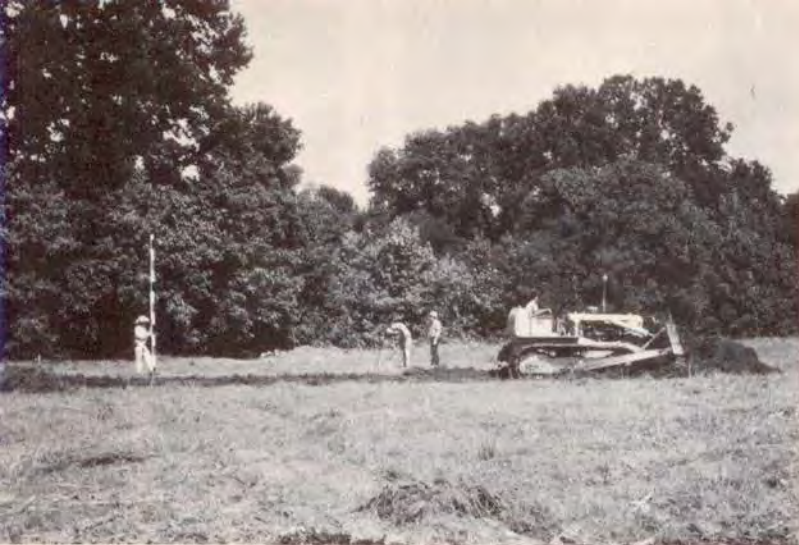
Detailed contour mapping of the site was made by rod and plane table methods in 1962 before the extensive bulldozing of the sites was commenced. The bulldozers were used to remove the overburden which covered the bone layers.
