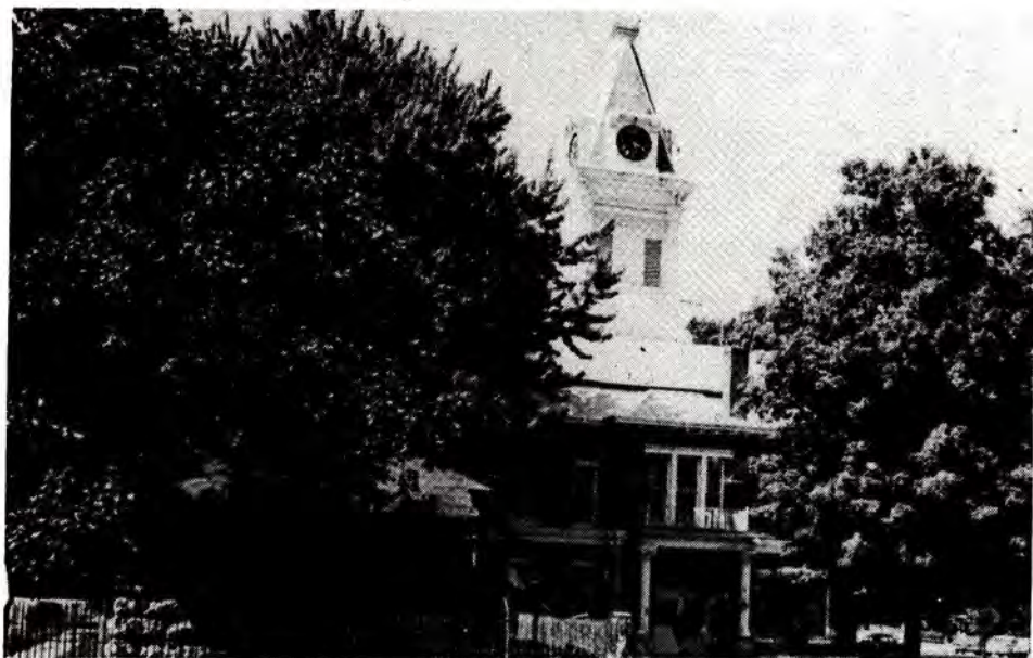
Carroll County's fourth Courthouse was built in 1884 at a cost of $16,437. During the 1937 flood, Coast Guard boats passed through the lower hall before the water got too high for them to go through the doorways.
