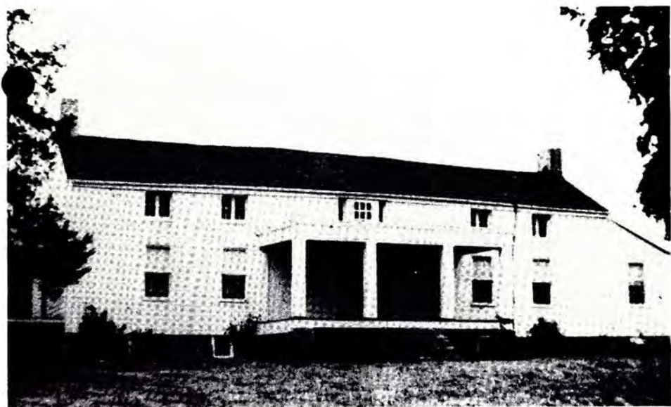
One of the best log houses in this part of the country is Grass Hills, located off Interstate 71. It was built in 1823 by Lewis Sanders, who brought the first pure bred cattle from England to the Ohio Valley in 1817.
